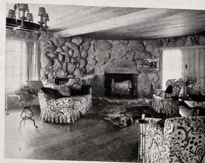
2. (Above)—Note the wide oak boards of this extremely smooth floor. A few basswood beams support the wood ceiling.
