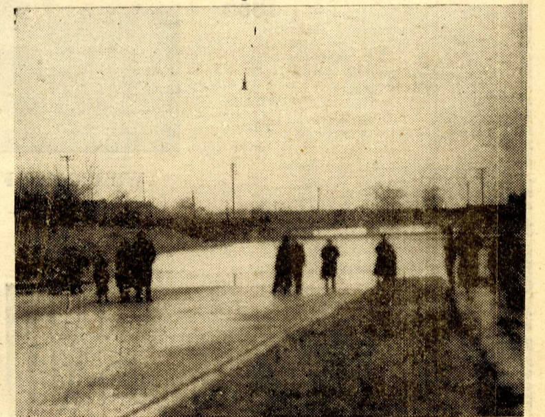
EAST SIDE TRUNKLINE sewers backed up, blocked the E. Maple viaduct with 11 feet of water. Firemen had to rescue several stranded motorists.
