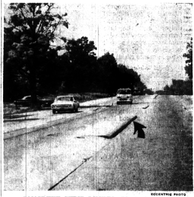
CONCRETE STRIP LINKED TO ACCIDENTS 3 vehicles crossed into oncoming traffic.
