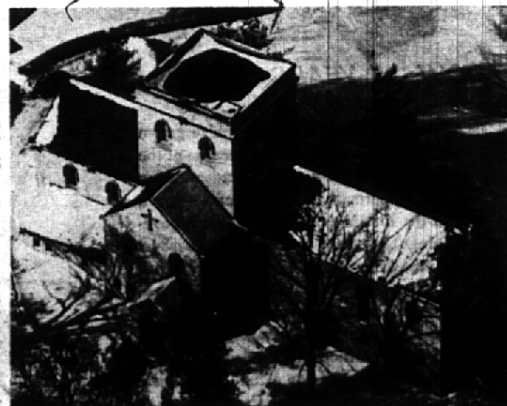
SOLE CATHOLIC CHURCH IN BLOOMFIELD HILLS Site was once the Stenycroft Estate.
