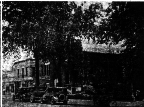
YESTERDAY'S CRAMPED QUARTERS Town was bursting at the seams.
