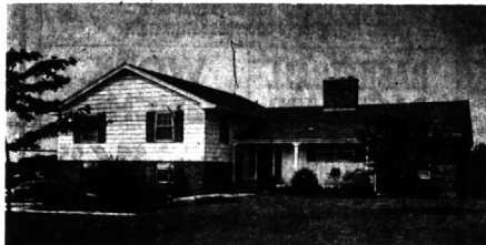
ULTRA SMART BRICK TRI-LEVEL — Eye catching appeal, both exterior & interior. Immaculate condition. Exquisite living room with brick fireplace. Formal dining rm. 20' family rm. Beautiful electric kitchen with built-ins and breakfast rm. Bloomfield schools. Attached garage; $38,900.
