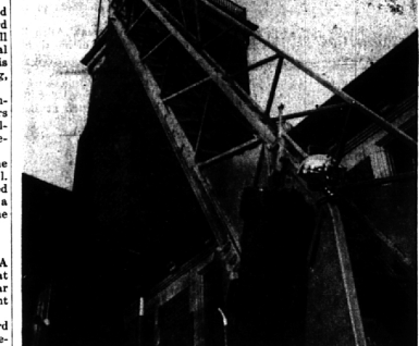
When Birmingham's municipal building chimney needed repairing this week, the fire department was pressed into service to aid in the project.
