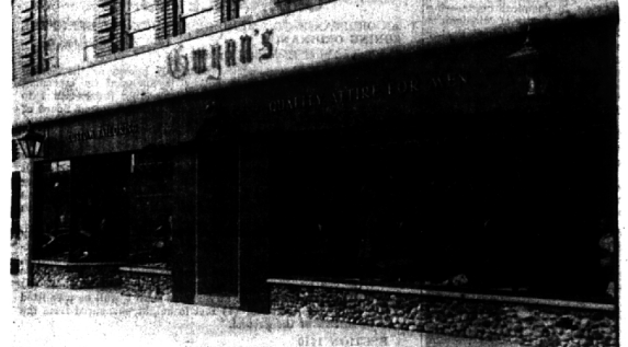
THE OUTSIDE OF Gwynn's men's store on S. Woodward has been entirely remodeled along with the interior. The project has more than doubled Gwynn's merchandising space. The store has been at location for nine years.
