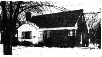
SPANKING NEW PAINT JOB—INSIDE AND OUT
