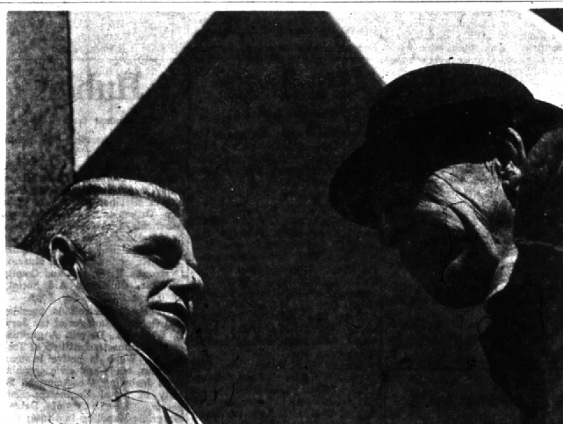
BIRMINGHAM BUILDING official Richard Schlosser (left) and his assistant, Frank VanFleteren, inspect and approve or reject all construction projects that are carried on within the Birmingham city limits. Here, the pair make a check of the new addition to Jacobson's store on W. Maple. All types of construction projects that cost more than $100 require a building permit under Birmingham law.
