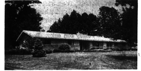
SPECIALLY CREATED HOME AT THE END OF A WOODED COURT. Four bedrooms (one ideal for in-laws), three bathrooms, large, deluxe "kitchen-family room" with fireplace and glass wall on to the patio. FULL BASEMENT. Convenient to all grades in new public and parochial schools.
