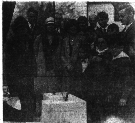
Laying the Cornerstone in 1929
