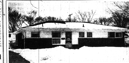
Well-planned Brick Ranch with slate entry, giving access to living room, Kitchen and/or Bedroom areas without "tramping" through other rooms. Many fine closets and storage areas.
