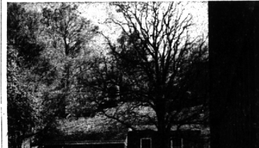
The century-old schoolhouse today. Wall of most recent addition is at right.
