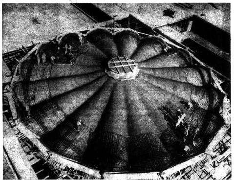
Twenty-five tons of cement were poured to make this thin-shelled roof over the library at the new Birmingham Wylie E. Groves high school. The architectural focal point of the building was designed by Linn Smith Associates, Inc., architects of the project. An additional nine tons of ce-
