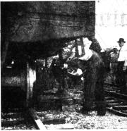
Operating one of the huge jacks which gradually lowered the car onto the wheel trucks, a woman completes the task. A train engine first was used to tow the runaway car task. A train eposition over the wheel trucks. Following the accident, the car had landed with one corner dug into the sod, the opposite end 10 feet into the air. The righting
