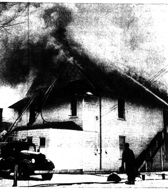
Smoke billows from Franklin's historic Community hall, 51-year-old landmark which was gutted by fire Monday with a loss estimated at $12,000. Nine pieces of fire equipment from four departments fought the blaze, shown here
