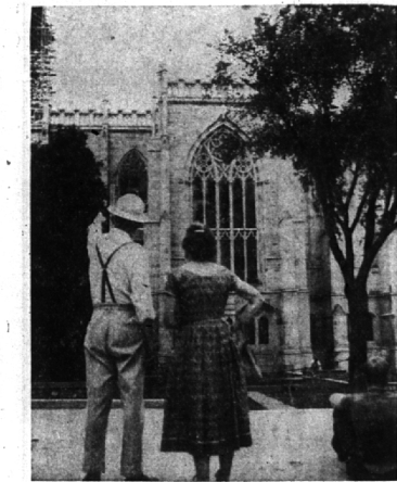
POINTING OUT the damage to a neighbor whose residence adjoins the Kirk in the Hills, construction Superintendent Robert Peden surveyed the still smoldering edifice at 5 p.m. the day after the fire. Dark spots in windows indicate where firemen broke glass to reach flames. At right is the Kirk minister's son, David DeWandt, resting after joining in the clean-up work in the undercroft.
