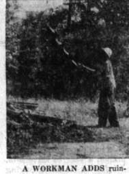
A WORKMAN ADDS ruined oak beam to burning pile outside the church on W. Long Lake road. Most of the delicately hand-carved oak ceiling beams were destroyed in the million dollar fire.
