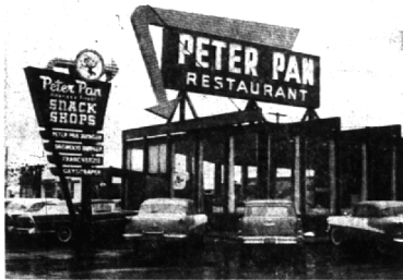
THIS NEW SIGN over the Peter Pan restaurant at Telegraph and Maple roads weighs over 3,000 pounds, measures 10 feet in length and has approximately 1,500 flashing lamps. One of the largest signs to be installed in one piece in the midwest area, it can be seen for two miles to the south and about one mile north of the restaurant.
