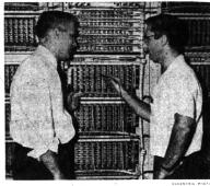
MAKING A LEAD test on the newly installed circuits are George Balligan, job supervisor of Western Electric, and Norman St. Onge, installer. The test instrument is placed at different sections where a whistle sound denotes proper hook-up.
