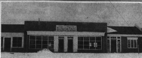
EXTERIOR VIEW of the Country Market which is located on the northwest corner of Southfield and 14 Mile roads. Scheduled to open about April 10, the new market will feature the finest meats, groceries and farm fresh produce.
