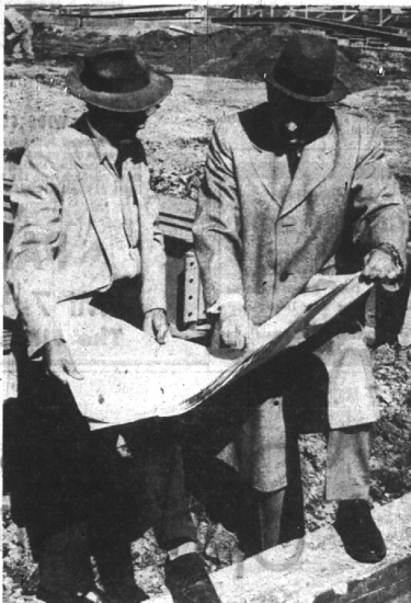
T. F. WALKER , right, 1042 Puritan, Birmingham, executive vice-president of Kent-Moore Organization, Inc., of Detroit, engineers and manufacturers of automotive service tools and equipment, goes over plans with construction supt. J. P. Whisman for Kent-Moore's new research and sales office now under construction in Warren township.
