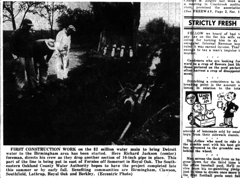
FIRST CONSTRUCTION WORK on the $2 million water main to bring Detroit water to the Birmingham area has been started. Here Richard Jackson (center) foreman, directs his crew as they drop another section of 16-inch pipe in place. This part of the line is being put in east of Fernlee off Somerset in Royal Oak. The South-eastern Oakland County Water Authority hopes to have the project completed late this summer or by early fall. Benefiting communities are Birmingham, Clawson, Southfield, Lathrup, Royal Oak and Berkley. (Eccentric Photo)
