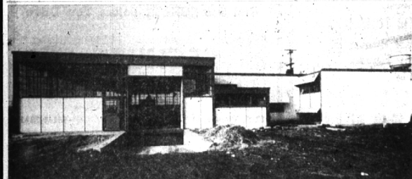
CARGILL OF DETROIT corporation, 2254 Cole, recently completed an addition to its factory floor space with 3,100 square feet, doubling the previous factory floor area. In announcing the completion of the addition, company officials also stated that an office expansion program would be started in the spring for the automatic machinery firm. Although only 2 1/2 years old, Cargill already produces automatic machinery for many of Detroit's leading automotive industries. Two additions at the far left and right in the picture flank the original size of the company's building.
