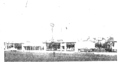
No. 1 Store 13520 Grand River Avenue, Detroit Over 10,000 square feet of floor space stocked with hardware, builders' supplies and home supplies.
