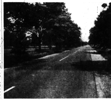
FOUR-YEAR OLD STRETCH OF SOIL CEMENT PAVING McKinley road north of Flushing handles 1,300 vehicles daily.
