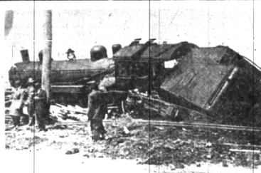
RAILROAD OFFICIALS SURVEY WRECKAGE Tracks were alongside 2-lane Woodward Ave.
