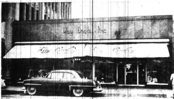
THE NEW front of the Kay Cooley Shop, 150 W. Maple, Birmingham, which has been remodeled inside and out. A 2 1/2 by 60' addition was added to the old store along with new fixtures, lighting and carpeting in both the old and new sections of the shop. This is Kay Cooley's 14th year in Birmingham.
