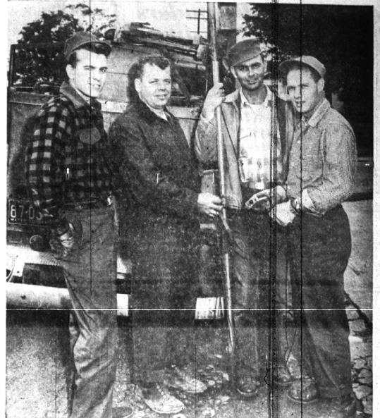
PART OF THE 330-MAN task force dispatched to New England by the Michigan Bell Telephone company to help restore that area's storm-mangled telephone service were these local area men. Shown at Augusta, Maine, are, from left, Lee Heimbecker, Birmingham; Jim Cappell, Birmingham; Harry Hammond and Charles Davis, both of Pontiac.
