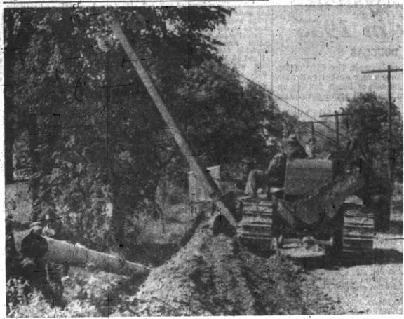
WORKMEN HURRY THE COMPLETION of Consumer Power company's 12 inch gas line through Troy township so that the line may be finished between the company's Adams regulator station north of Auburn road and the Coolidge plant at Fourteen Mile road and Coolidge within this year's building season. Workmen are pictured above laying the large pipe parallel to Coolidge road south of East Long Lake road in the north Adams section of Troy township. Use of the pipe line will bring an additional supply of gas into the Coolidge road plant for South Oakland County customers. (Eccentric Photo)
