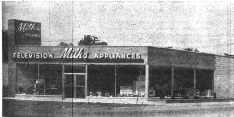
As you can see from the above photo our new store takes advantage of the best that modern architecture has to offer. No expense has been spared to present to you the public a store that is easily reached and identified, and designed to facilitate the wisest choice of appliances as seen by abundant natural light coming through the large, store front windows.
