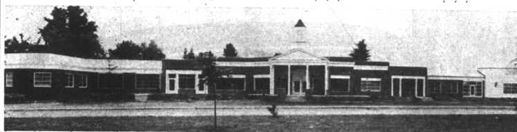
NEW PONTIAC-CADILLAC AGENCY BUILDING AT SOUTHEAST CORNER WOODWARD AND MANOR ROAD
