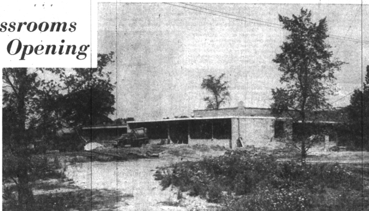
TO GET AN OVERALL picture of the Pembroke elementary school, the photographer really needed (but didn't have) a helicopter. The 13-classroom school is laid out in three wings to assure pupils of ample natural light and ventilation. Workmen are going to be pressed to have this school open for use by the September 7 deadline. (Eccentric Photos)
