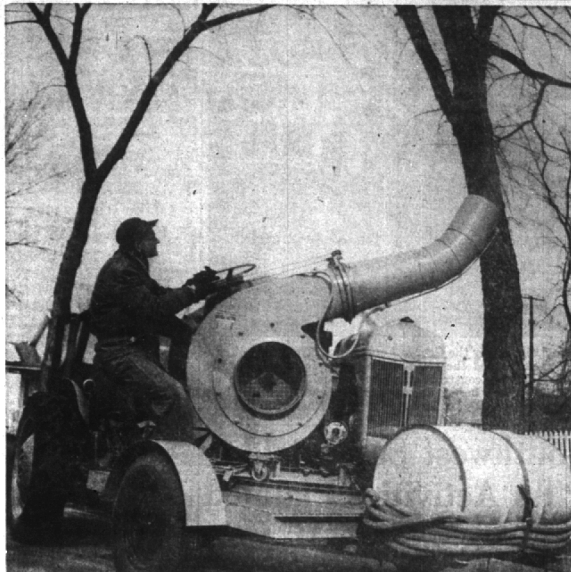
BIRMINGHAM'S NEW "MIST TYPE" TREE SPRAYING MACHINE Paul Breniser directs DDT fog on elm tree on Webster street. (Eccentric Photo)
