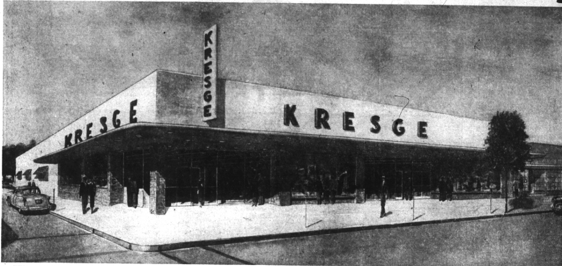
THIS IS KRESGE COMPANY'S NEWEST STORE. A HALF-MILLION DOLLAR BUILDING ON SOUTHWEST CORNER OF W. MAPLE AND HENRIETTA Completely airconditioned and modernly lighted, it has been specifically designed for the latest in customer convenience
