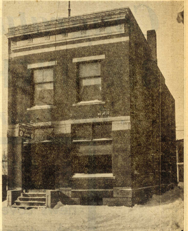
ABOVE: FORMER EXCHANGE ON PIERCE ST.
