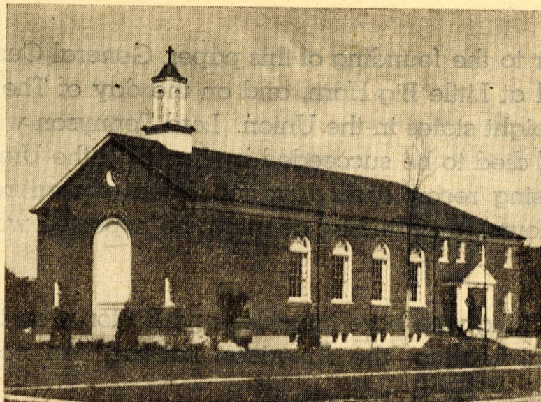
TOWNSITE COMMUNITY CHURCH Congregational church situated on Southfield road
