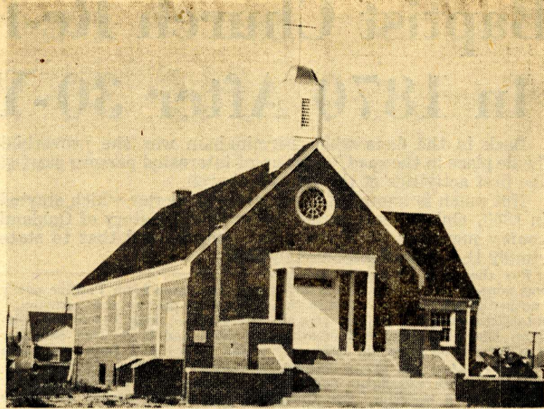
CONGREGATION'S NEW CHURCH ON 14 MILE RD. Former location was on Bennaville near Woodward
