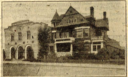
Detroit Chapel—now 3975 Cass Ave.
