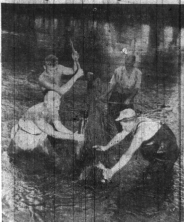
Conservation department crews will be busy again this year improving some of Michigan's lakes and streams. The work includes a variety of activities, such as placement of small dams and deflector logs, planting of erosion stopping growths and pollution control. Here a crew, working on the North Branch of the Au Sable plants a "digger" log. The current will move around the log and dig deep fish pools in the stream bed.
