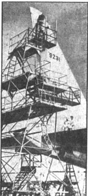
TALL TAIL—It's no tall tale when mechanics working on this highly secret eight-jet bomber in Seattle say the huge ship is "way up there" even when it's on the ground. Special scaffolding is needed to permit adjustments on the 48-foot-high vertical tail.
