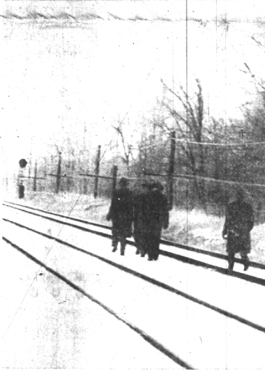
... ALONG A HALF-MILE STRETCH, the four men closely inspected the fencing so they can more intimately know the problem and better report to top GTWRR management possible corrective measures that might be taken to sharply reduce or even eliminate the hazards that have arisen. Marquess said it would be several weeks before the railroad would be able to announce its decision. (Eccentric Staff Photos)
