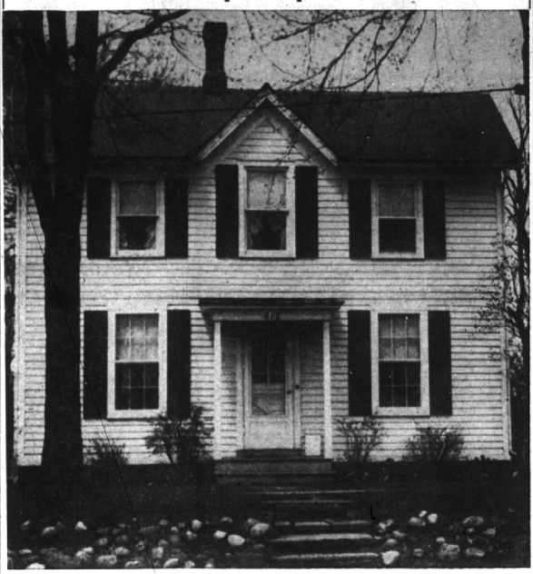
ONE OF BIRMINGHAM'S OLDEST HOMES IS 412 WILLETS. Elijah Willets built this frame house in 1821. (Eccentric Staff Photo)
