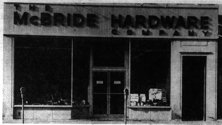
MODERNISTIC, NEW FRONT OF THE McBRIDE HARDWARE COMPANY AT 154 SOUTH WOODWARD Grand opening in new location to be Friday and Saturday, March 28 and 29
