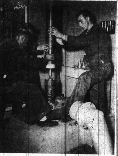
A NEW SECTION OF PIPE IS CAREFULLY LOWERED to meet a second section previously dropped as Firemen M. Harper, Asst. Chief Pork Smith (hidden behind Harper), and George Wallace get set to join the two. Three pumps in the city were given major overhauls within six days as firemen worked night and day to save the city's dwindling water supply. (Eccentric Staff Photos)
