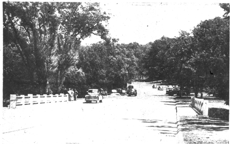
WORKMEN HURRIED COMPLETION OF THE WEST MAPLE widening and residents praised the straightening of the roadway to cross the new four-lane bridge which re-
