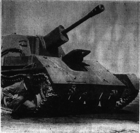
A CAPTURED SOVIET-MADE TANK is inspected by a Birmingham serviceman, Sgt. Leonard Bailey, at the Aberdeen (Md.) Proving Ground. The picture of the SU-76 self-propelled gun was taken by Ed Wergelke and appeared in the April 14 issue of NEWSWEEK which described the tank as being "a good anti-personnel and anti-tank gun mounted on a poor chassis, too cramped for the crew, too lightly armored with crude welding that, when hit, splits like a seam."
