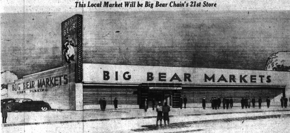
Construction work began this summer on the $220,000 building which will be the Big Bear market here. This store which will be located at the corner of Woodward and Sheffield will be the Detroit chain's 21st store. The off-street parking lot will accommodate 175 cars.
