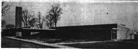
FRONT VIEW OF TORREY SCHOOL BUILDING Site is bounded by Torrey, Lincoln, Eton and Humphrey streets.
