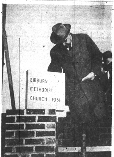
CORNERSTONE CEREMONIES for Embury Methodist church, located on 14 Mile road were held Nov. 11. Here Dr. William E. Harrison, district superintendent, applies the first trowelful of cement prior to the setting of the stone. Pastor of the church is the Rev. Reginald Becker.
